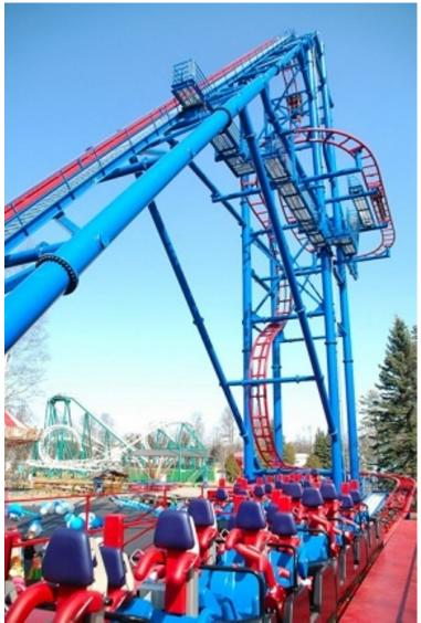
Lifting of 1 vehicle with an electric motor at 27 meters height, chute by gravitation
